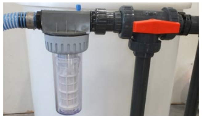
Heavy duty filter and 3-way valve
