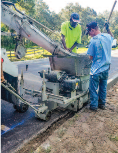
The front wheels of the 150 can be shifted to allow the machine to pour over a trench.
