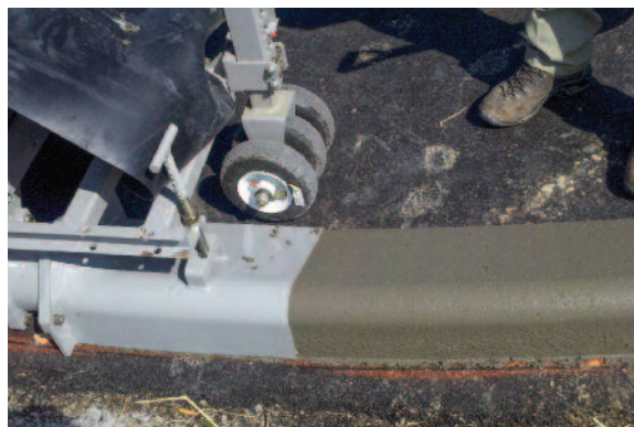
Using a chalk or paint line on the ground as a guide, the operator has a clear view of the path in front of the machine.
