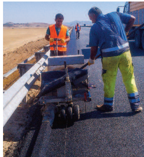
The 150 is easy to operate; one person steers while another ensures that the concrete or asphalt is reaching the auger.
