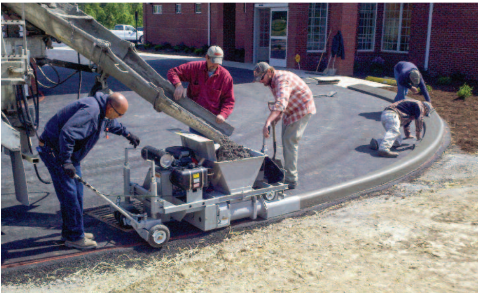
The extrusion process propels the machine forward.
