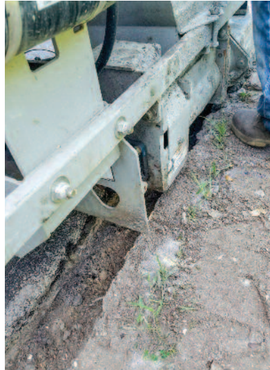
Trench curb can easily be poured with the 150 extruder.
