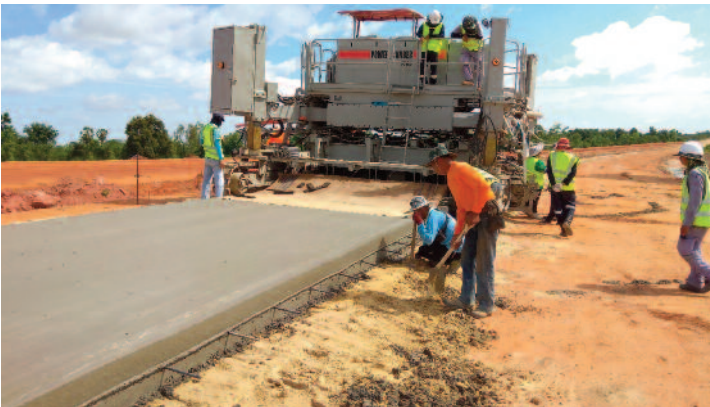
▲ Power Curbers 7700 Multipurpose Slipform Machine Paving
