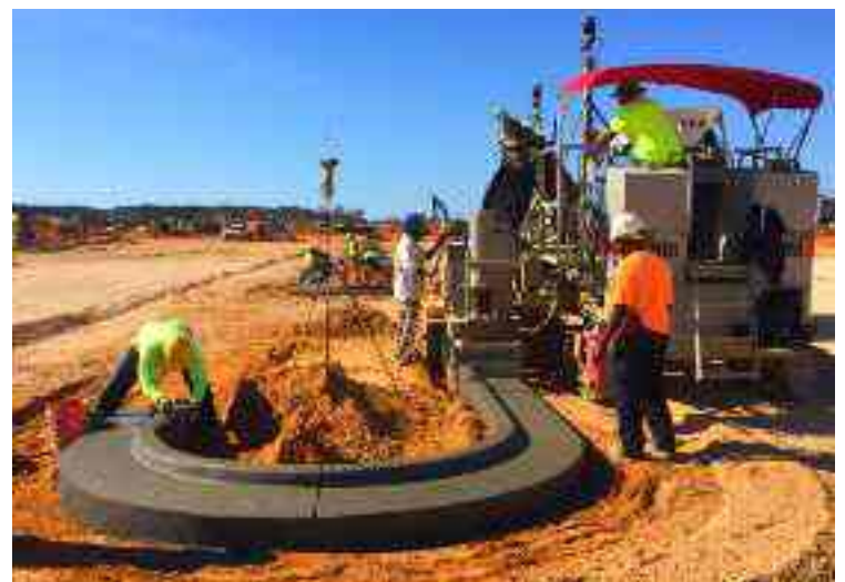
Pouring curb & gutter with 3-D (stringless) control.
