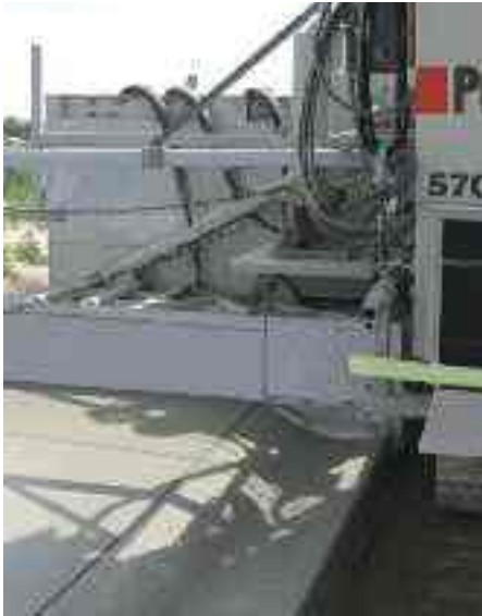
Monolithic curb, gutter, and sidewalk.
