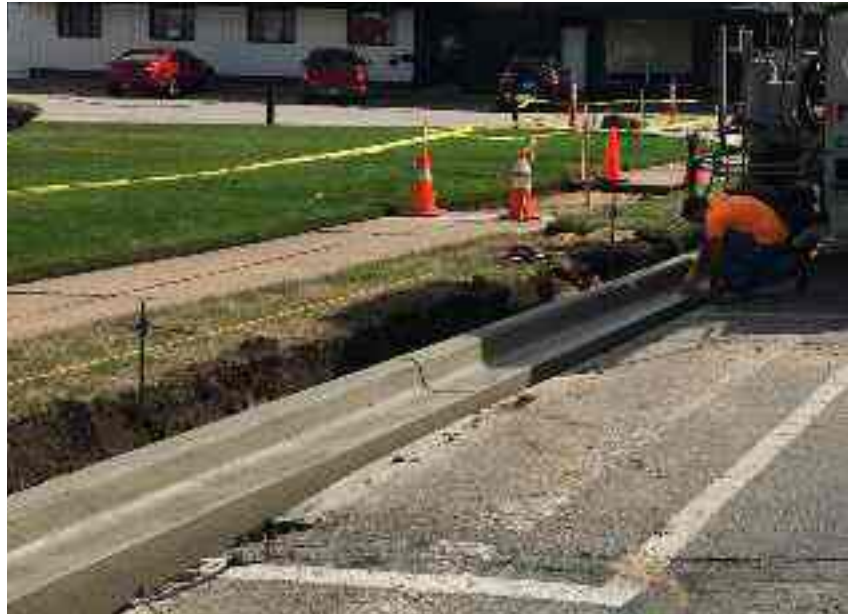
Curb & Gutter in a rehab application
