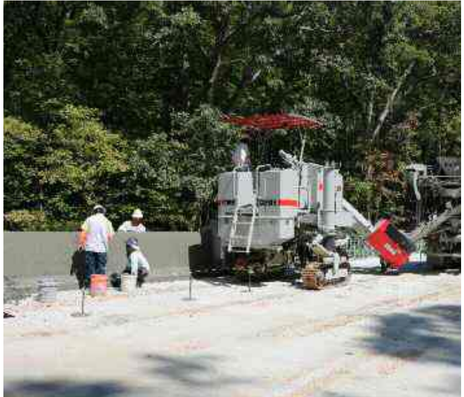
5700-D-MAX pouring bridge parapet over reinforcement. Includes optional canopy.
