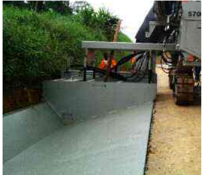
V-Ditch in Equatorial Guinea, 7' (2.2m) wide and 18" (.45m) deep, poured adjacent to pavement.
