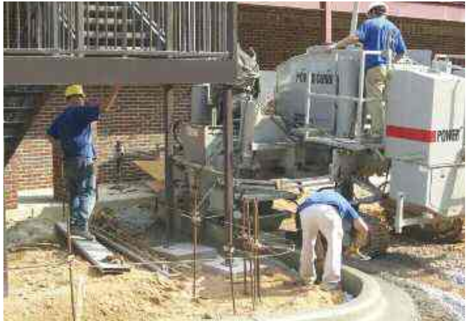
Machine maneuvers in tight areas, minimizing tie-ins.
