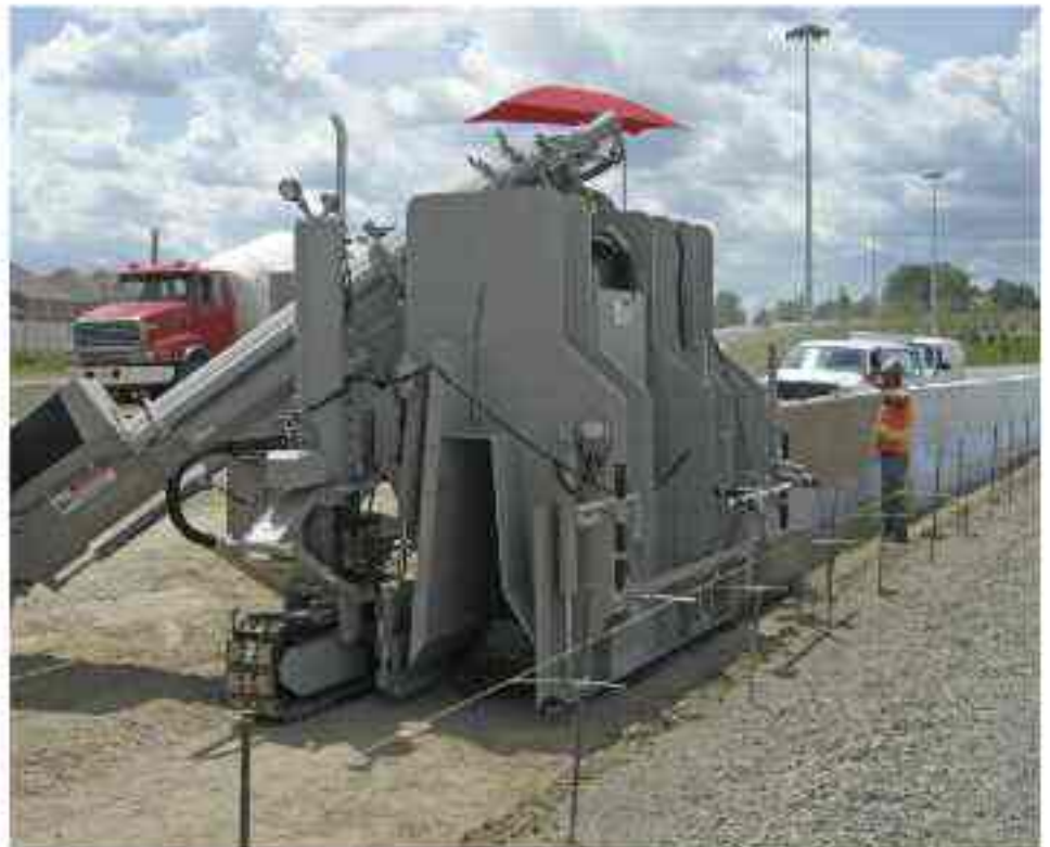
MAX package pouring large variable barrier wall.
