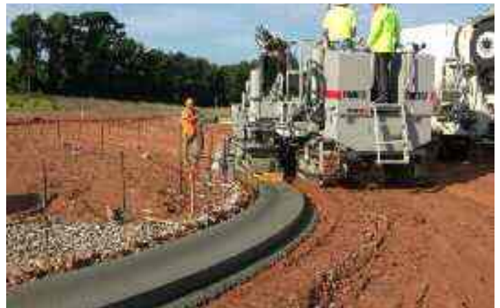
The rear post on the 5700-D-MAX can be returned to its standard position for pouring curb and gutter.
