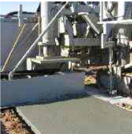
Sidewalk adjacent to back-of-curb. Sensing off-curb.
