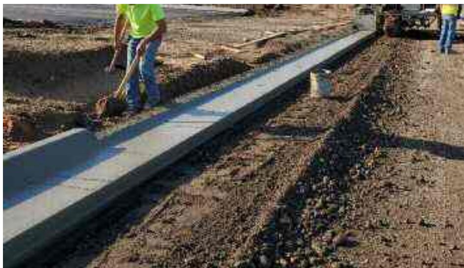
Driveway knives reduce wasted material and labor. Some hand finishing is required.
