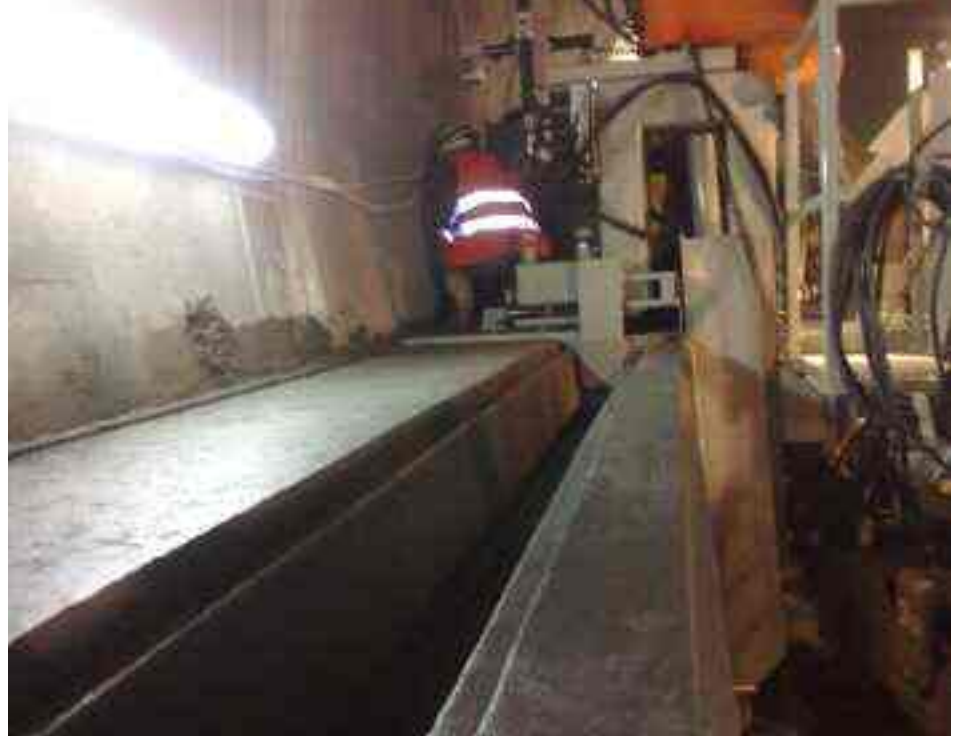
Platform & wall structure poured along a tunnel wall in Turkey – mold is adjustable in height and width to accommodate varying tunnel diameter.
