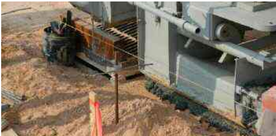
Trimmer lifting over catch basin to pour the curb as closely as possible.
