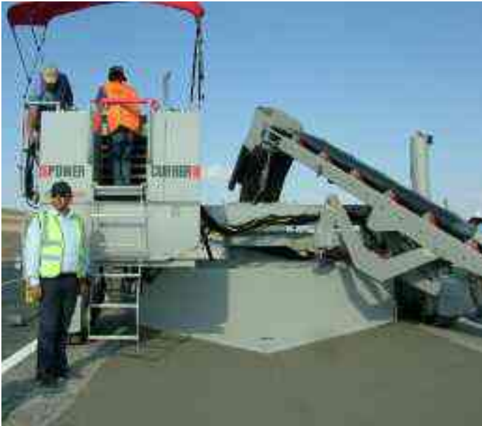
Ditch Liner in Turkey, 12.5' (3.8m) wide and 2' (.6m) deep, adjacent to pavement on both sides. (shown with custom belt conveyor)
