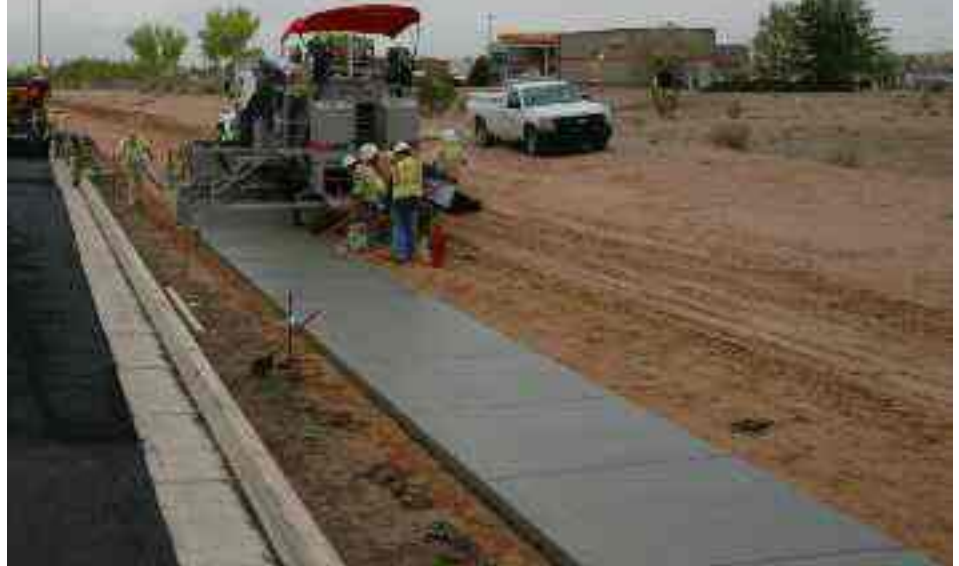
Pouring a 6' sidewalk.
