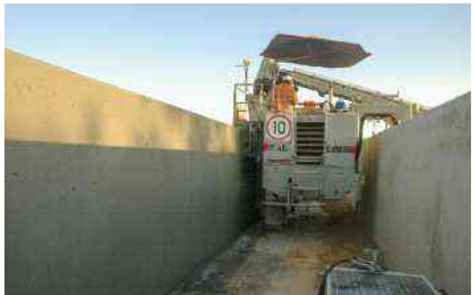
Canal in Australia, base 12' 5.5" (3.8m) wide and sides 6' 10" (2.1m) high. (Shown with custom belt conveyor)
