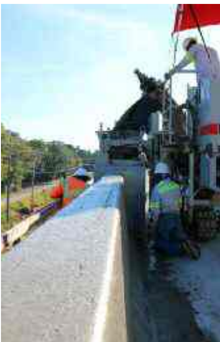
Close up of Bridge Parapet
