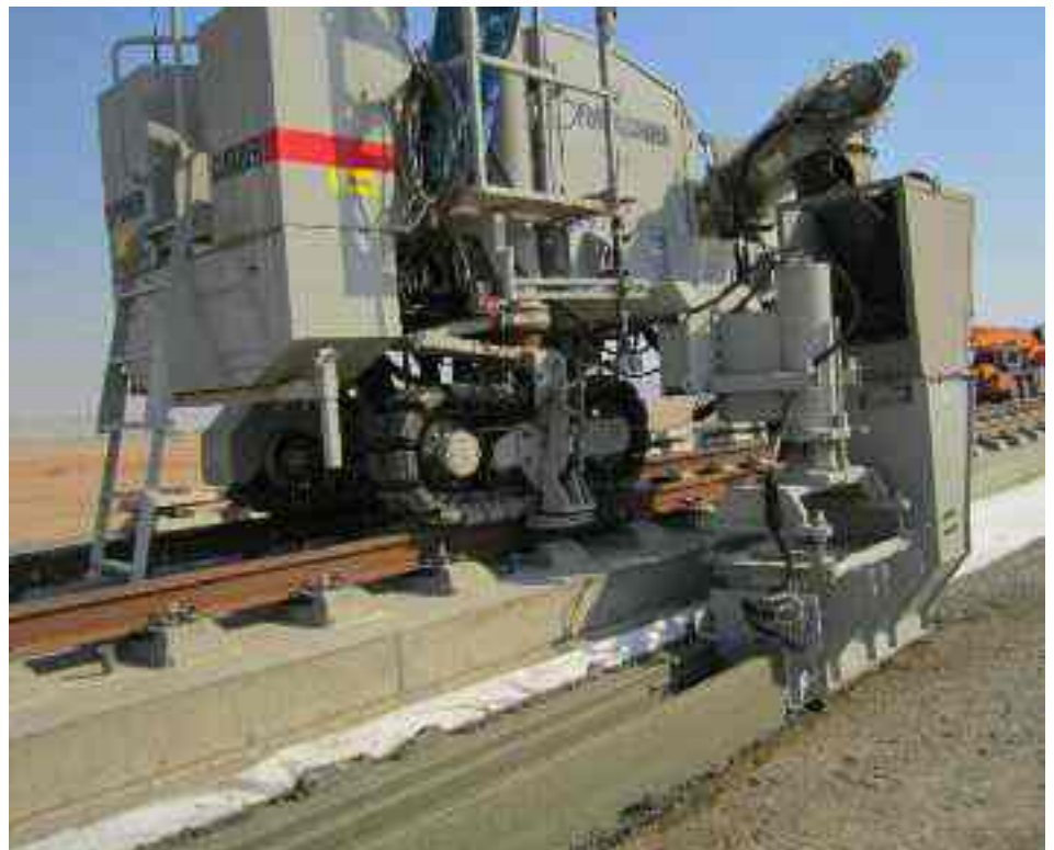
High-speed rail application in Saudi Arabia using custom rail attachments to pour a utilities trough.
